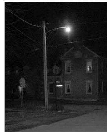
The above photo shows a Rocheport street light with the new LED light bulb. Though it's difficult to see the difference in light color, the even dissipation in the lighting is evident when compared to the high-pressure sodium light, shown at left.
