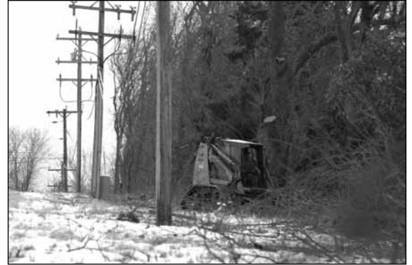
Right-of-Way Crews also clear the brush under power lines, creating a 15-foot path from the ground up.
