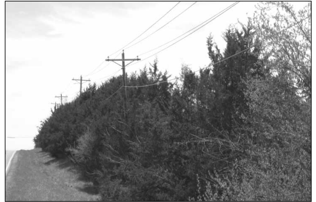
The trees under this three-phase distribution line (above) will soon be removed. Lines in this condition will take longer to restore following an outage. The tree at right was trimmed two years ago. However, fast-growing shoots have already grown past the height of the power lines.
