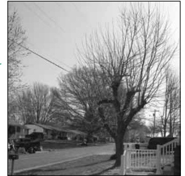
The trees under this three-phase distribution line (above) will soon be removed. Lines in this condition will take longer to restore following an outage. The tree at right was trimmed two years ago. However, fast-growing shoots have already grown past the height of the power lines.
